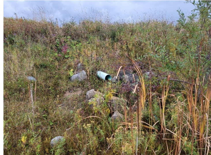
Image 2: Disturbances associated with previous construction grading activities.
