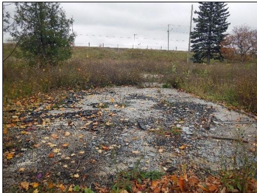
Image 13: Disturbed Concrete Pad & Former House Location (Facing S)
