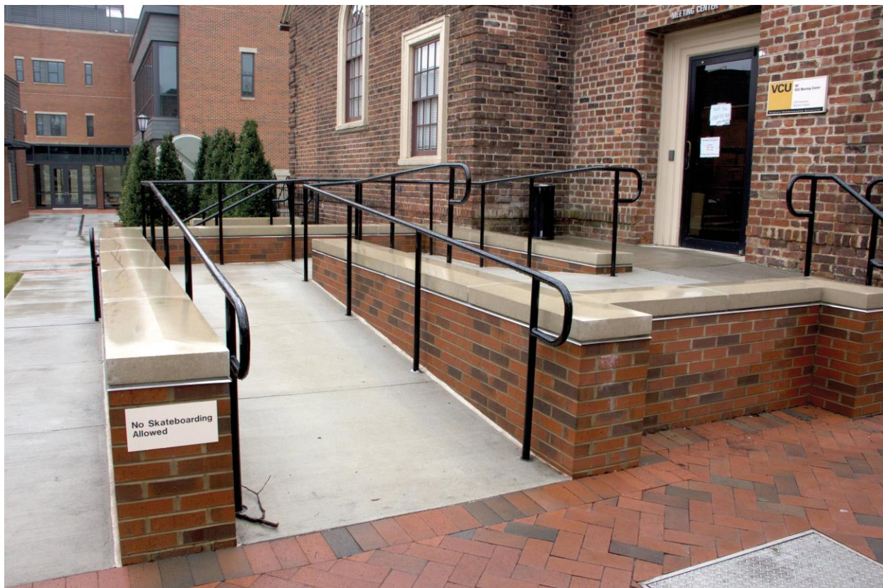
Image 3: Exterior entryway ramp.
