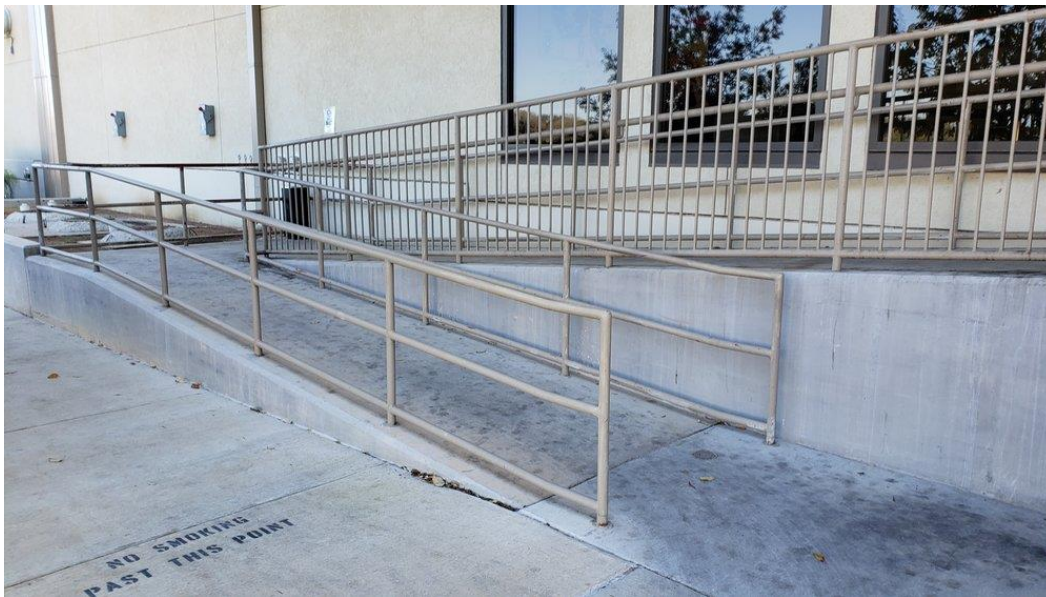
Image 5: Ramp guard & handrail.
