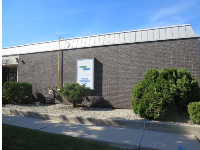
Richard H. Neath Water Treatment Plant
